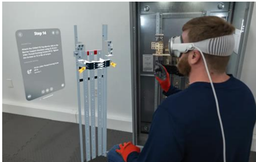
Figure 5. A man wearing an Apple Vision Pro next to a Siemens P5 power panel. He is looking at a digital overlay of BILT immersive instructions including a 3D rendering of the panel and a text window.
